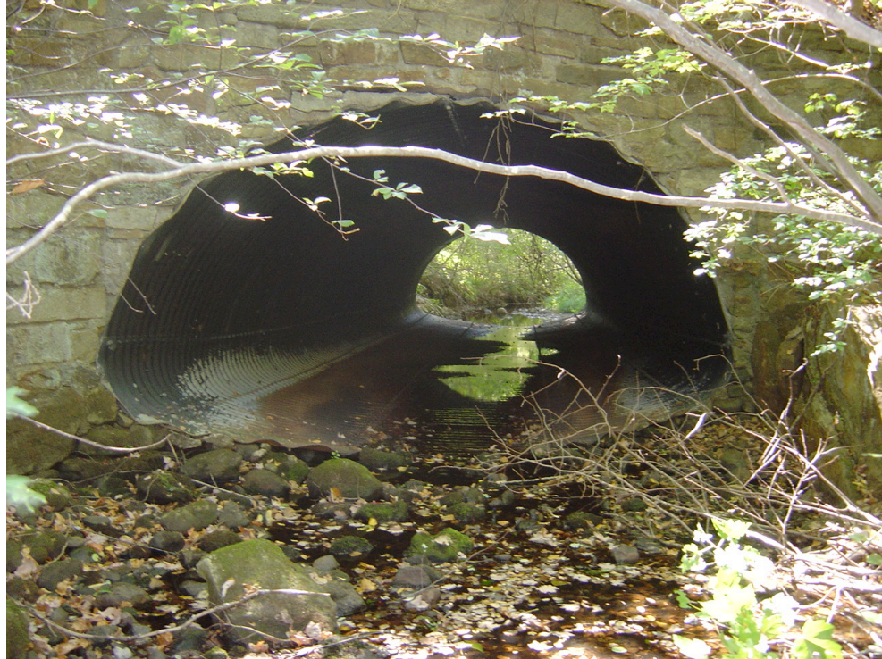
Figure 19. Culvert downstream of Site 5
