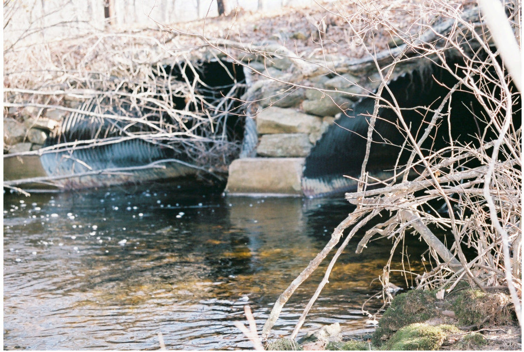
Figure 17. Culverts downstream of Site 4
