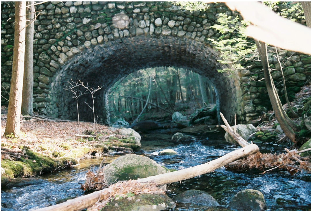
Figure 14. Stone bridge downstream of Site 3
