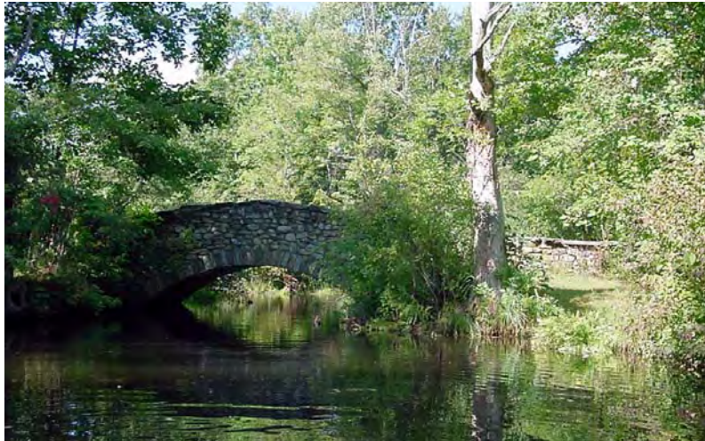
FIG 38. View of the Brook Bridge, 2004
