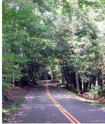
FIG 17. Typical Road in Watershed Smaller roads within the watershed are typically hilly, narrow, and windy, due to the rocky topography.
