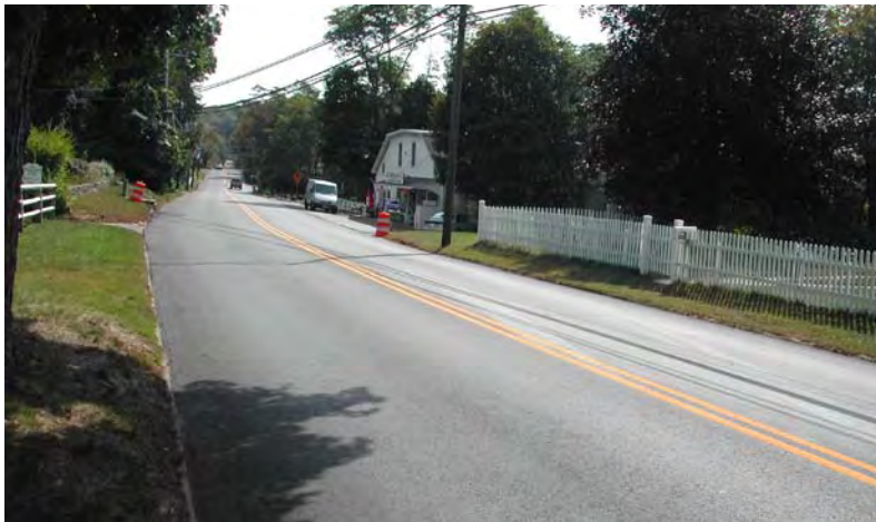
FIG 20. Route 156, Lyme Route 156 was recently repaved and widened.
