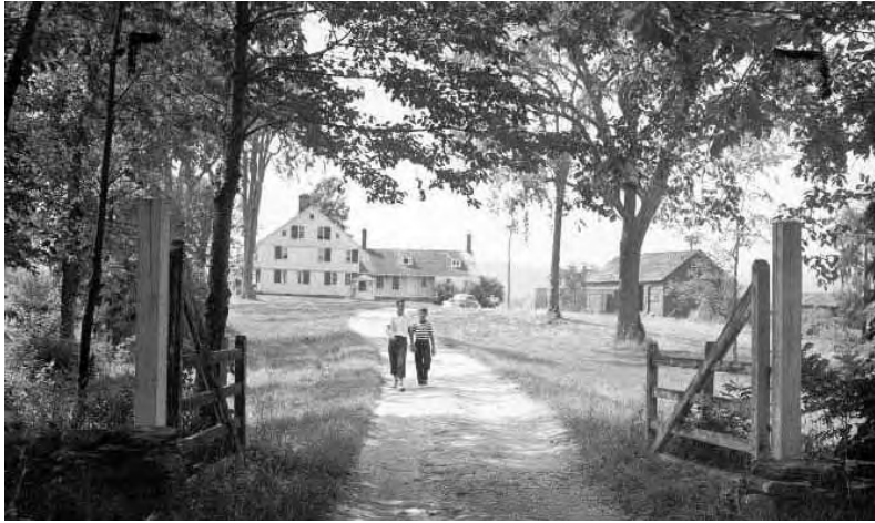
FIG 41. The Mumford House, 1945 View looking down the driveway of the Mumford house and farm, 1948.
