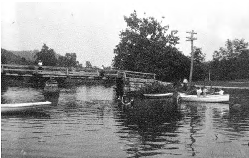
FIG 68. Hamburg Bridge Over Eightmile River, pre-1936 The former stone and wood structure of the old Hamburg bridge.
