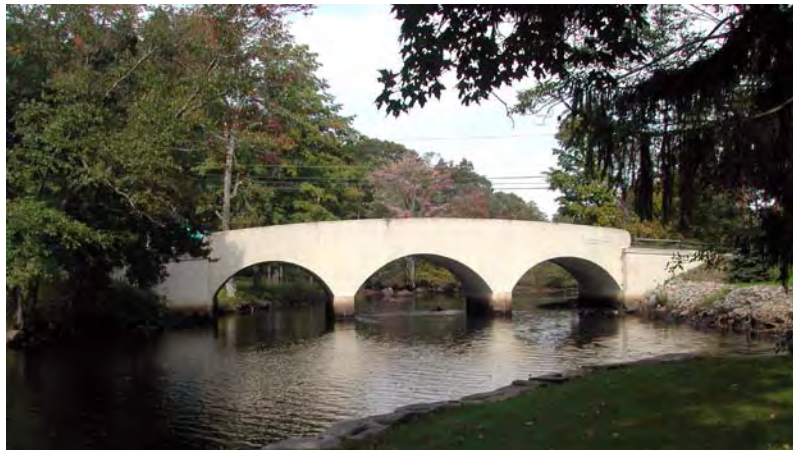
FIG 69. Hamburg Bridge Over Eightmile River, 2004 Replacement concrete bridge built by the Army Corps of Engineers in the late 1930s after the hurricane of 1936.
