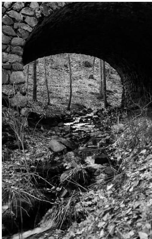
Stream Crossing in East Haddam
